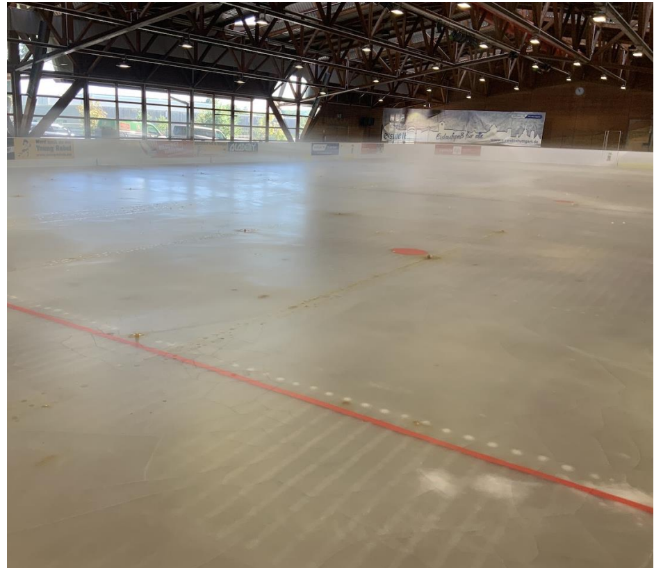
Formation of fog due to the ingress of warm and humid summer air
