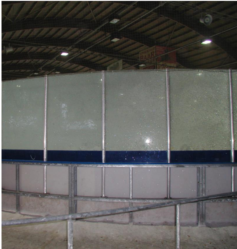
Condensation due to the ice rink being partially open
